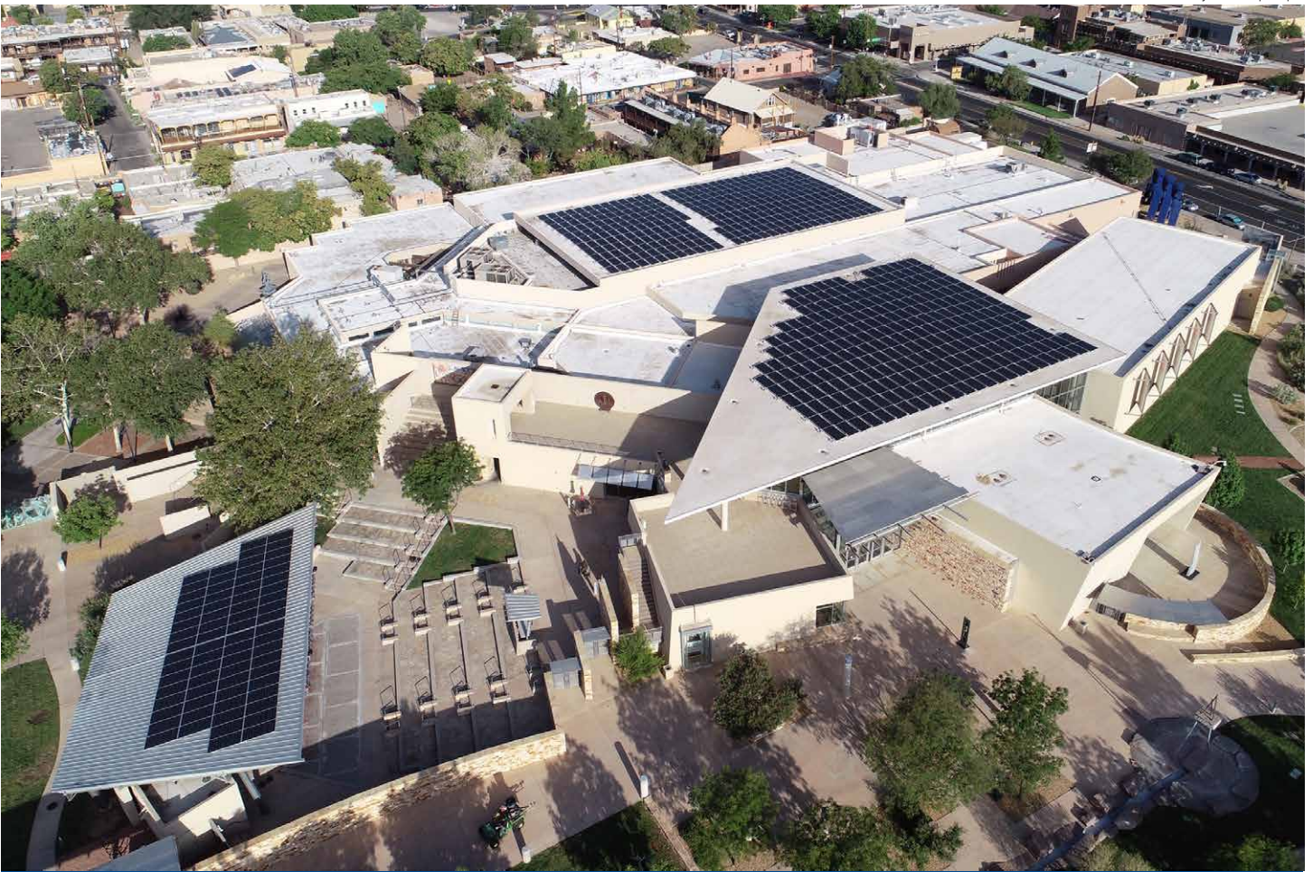
Rooftop solar panels on the Albuquerque Museum.
